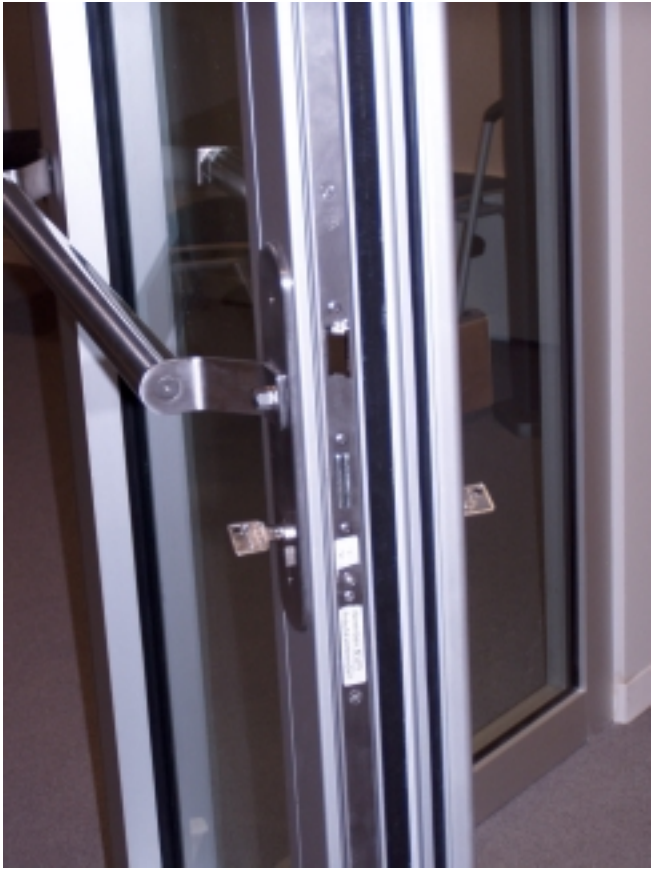
Multi-Point Locking Mechanism
